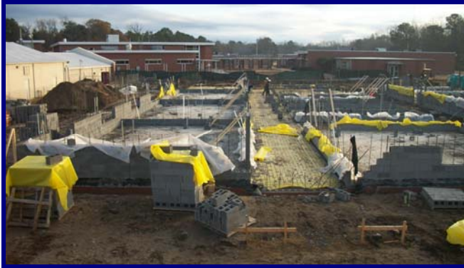
North Corridor, Floor Slab and CMU Walls
