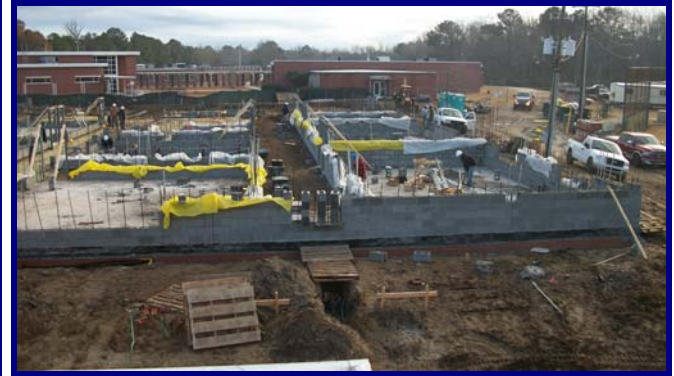
South Corridor, Floor Slab and CMU Walls
