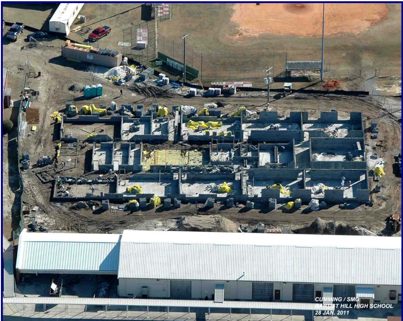
CMU Walls Installed to First Bond Beam Height
