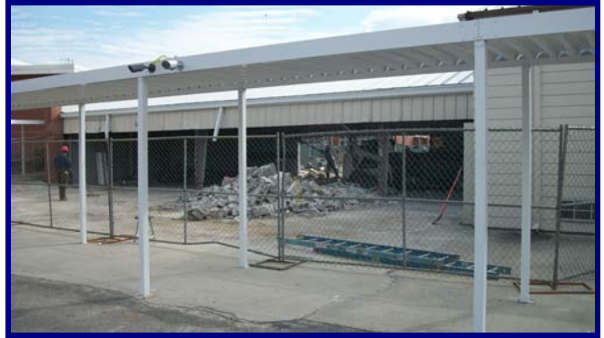
Demolition of Existing Weight Room Underway
