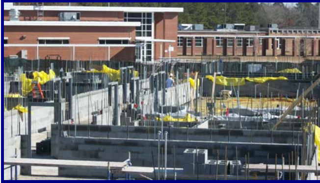
CMU Walls Installed to First Bond Beam Height
