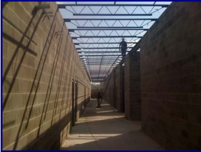
Roof Joist Steel Erection Complete at Corridor
