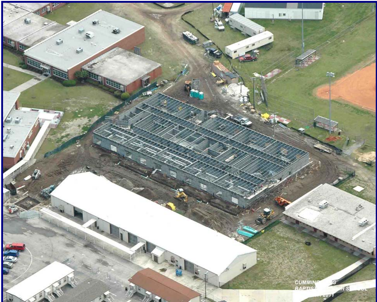
Roof Joist Steel Erection Complete at Corridor
