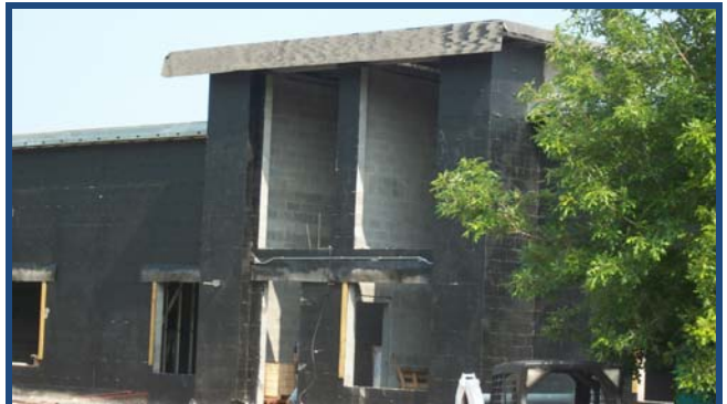
Exterior View of Southeast Entrance
