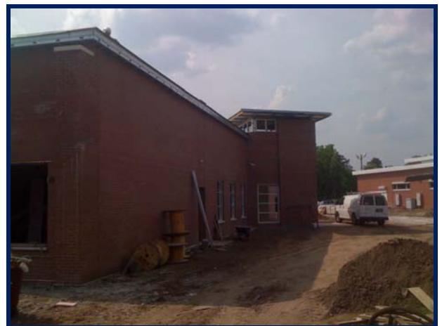
Exterior Brick Complete to Main Entry
