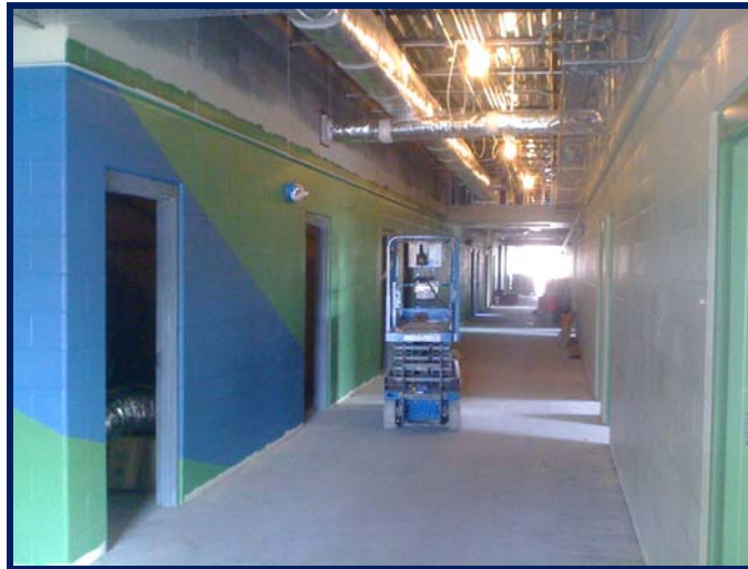
Interior Corridor With Finish Paint Underway
