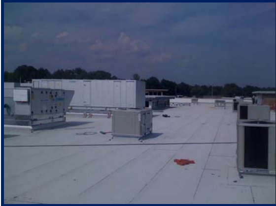
Roofing Complete with HVAC Units Installed
