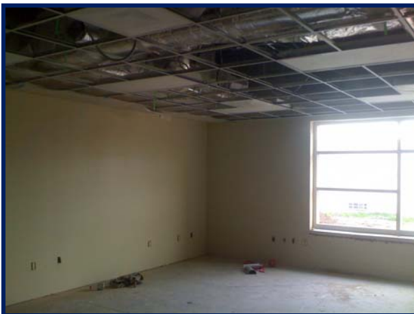
Classroom: Ceilings & Windows Installed
