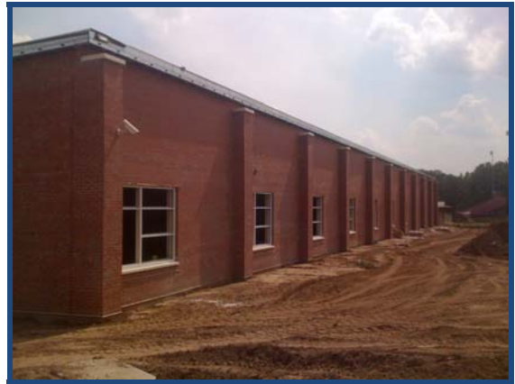
Exterior Brick Complete: Windows Installed
