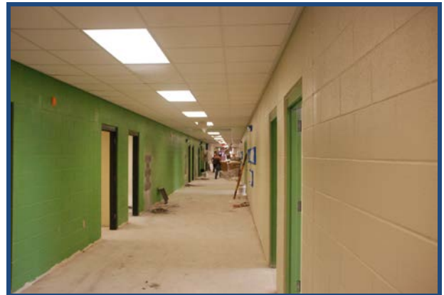
Main Corridor with Ceiling Installed
