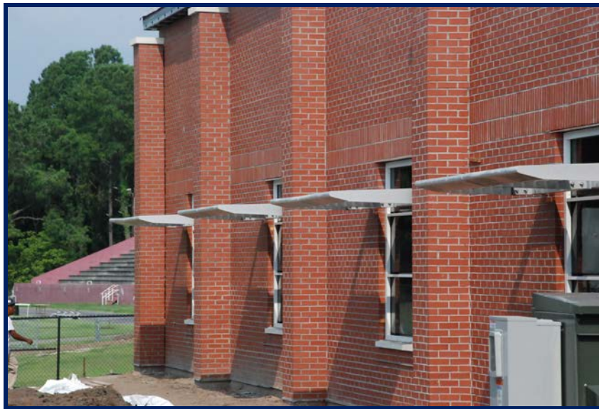
Exterior Brick Complete and Window Sunshades Installed
