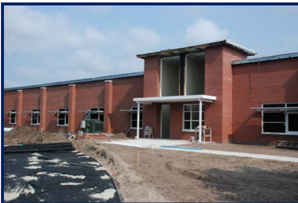
South Building Exterior at Fire Loop Road
