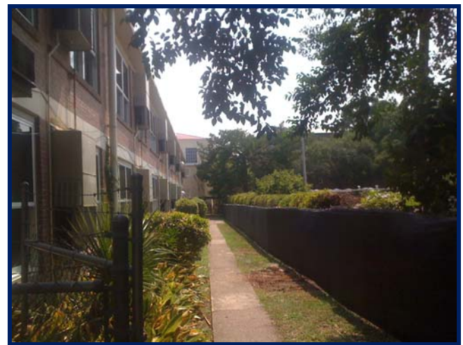
Fencing Installed to Protect Adjacent Properties and Historic Walls
