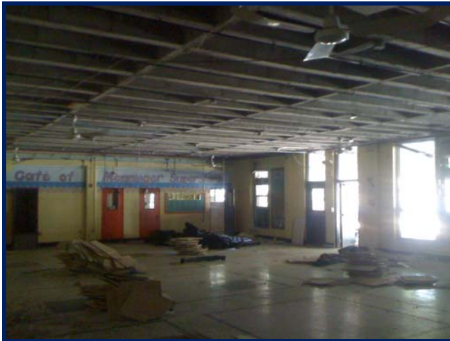
Cafeteria Ceilings Removed for Recycling
