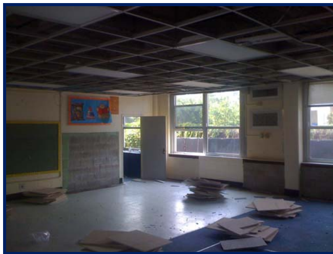
Demolition Underway at Existing Classrooms
