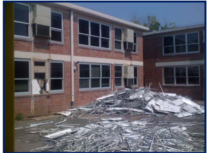
Obsolete Ceiling Grid and Lights Separated for Recycling
