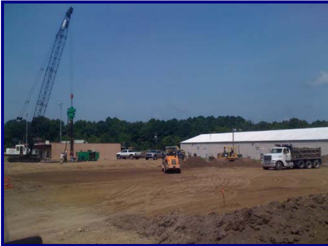
Earthquake Drain Installations Ongoing
