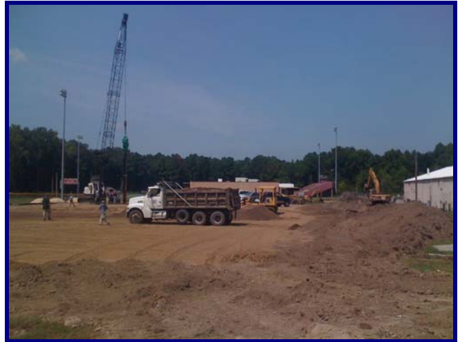
Fill Material Being Imported to Building Pad
