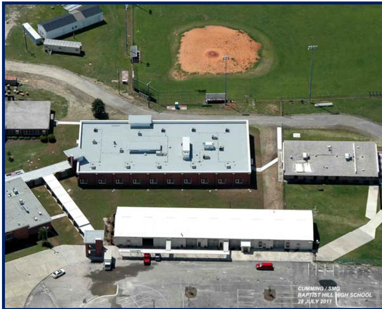
Latest Aerial Photograph
