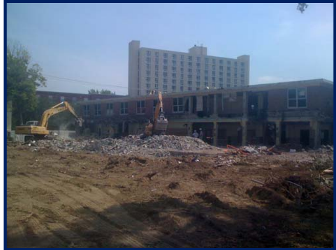
Kitchen - Cafeteria – Admin Area Demolition Complete
