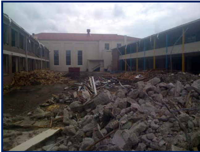
Demolition Progress – View through Courtyard towards Memminger Auditorium
