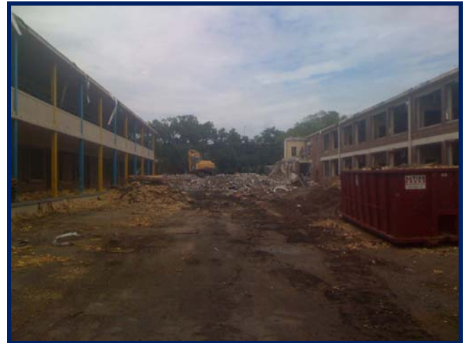
Demolition Progress – View through Courtyard towards Demolished Cafeteria
