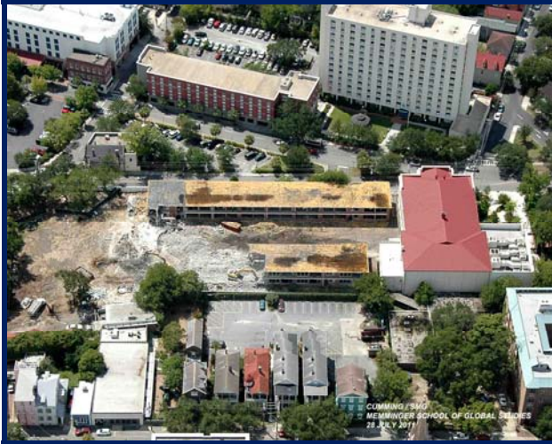
July 2011 Aerial - Cafeteria / Kitchen Demo Complete with North Wing Underway
