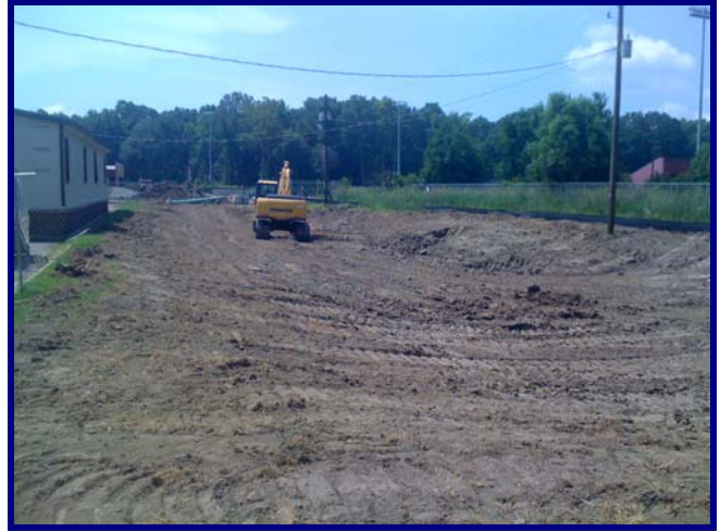
Water Retention Pond Construction
