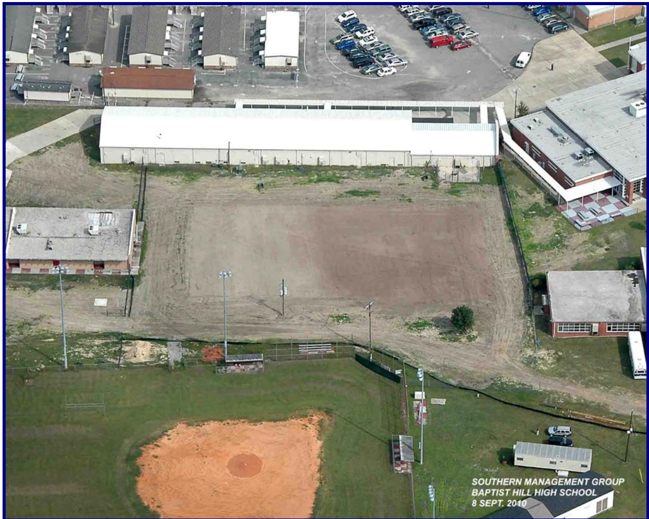
September 2010 Aerial Photograph – Building Pad Complete
