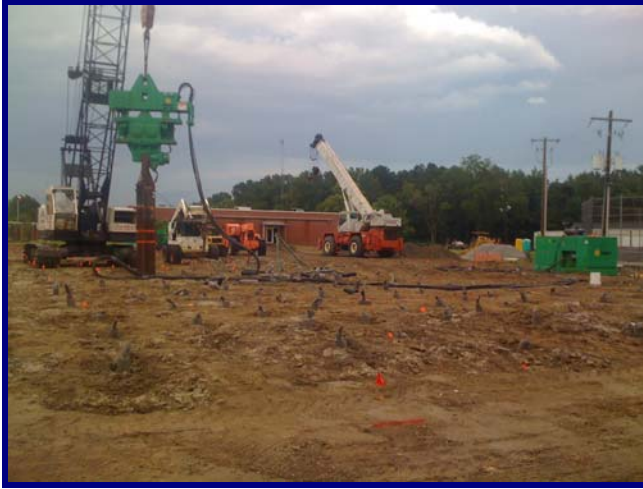
Earthquake Drain Installations
