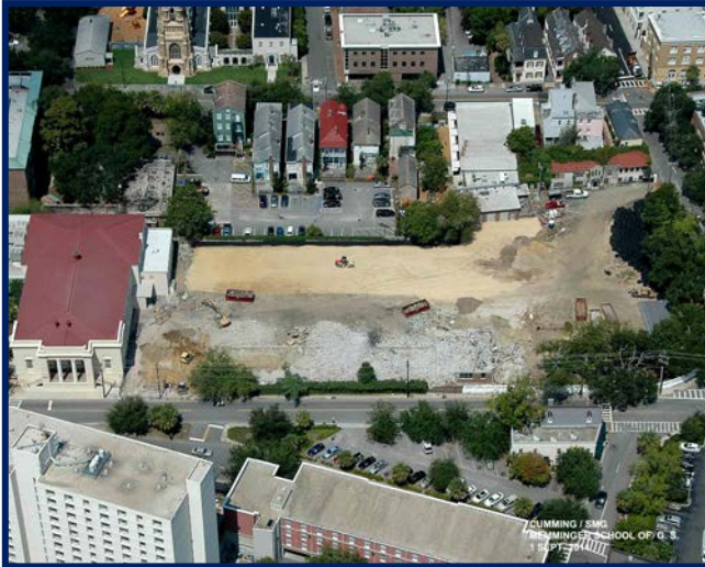
September 2011 – Aerial Photograph Major Building Demolition Complete
