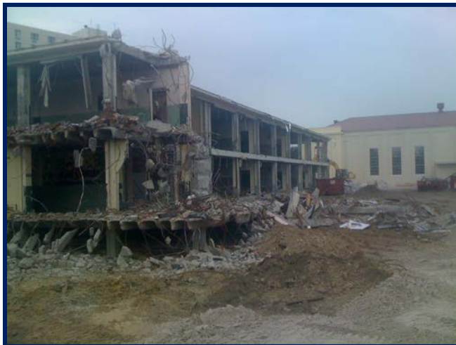
In Progress Photo of South Wing Demolition
