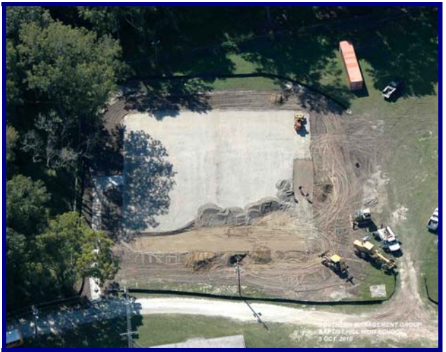
Tennis Courts Underway on Site by Others
