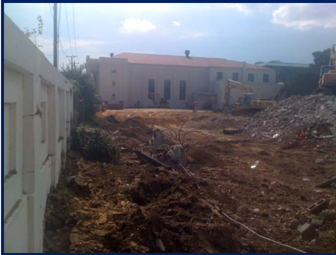
South Wing Demolition Complete with Final Removal of Debris in Progress
