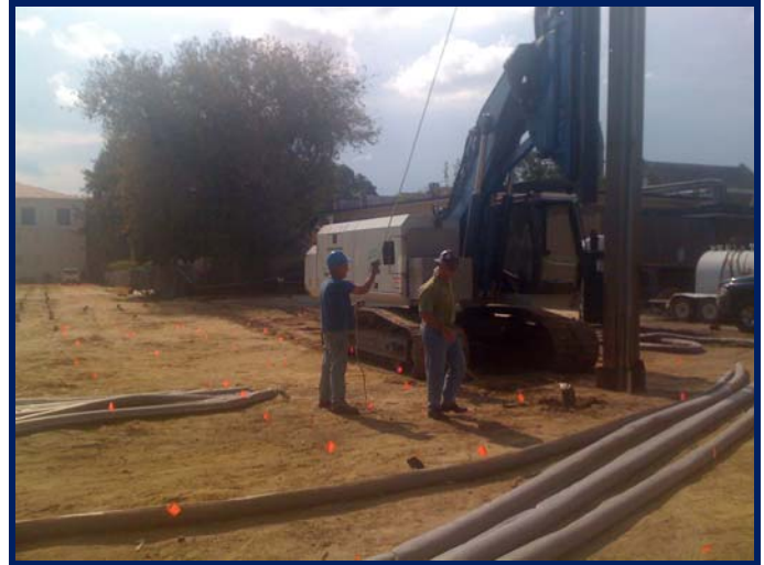
Earthquake Drain Installations Underway With Principal of Installation Company on Site
