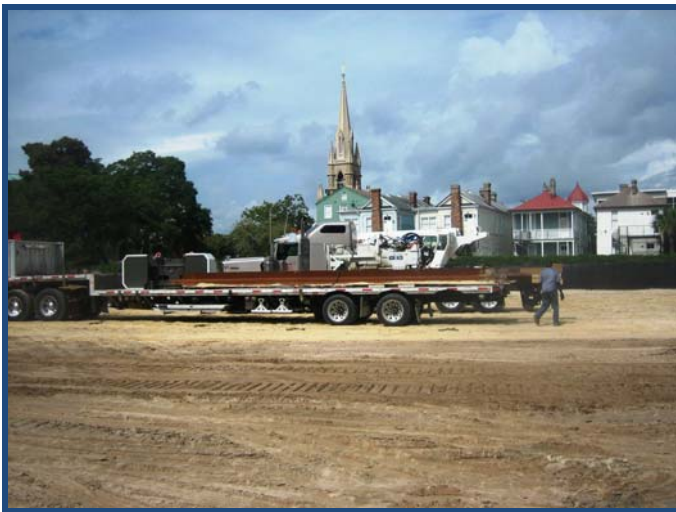
Earthquake Drain Installation Rig Being Dismantled after Completion of Drains
