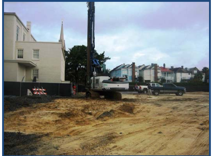
Final Earthquake Drains Being Installed Adjacent to Memminger Auditorium
