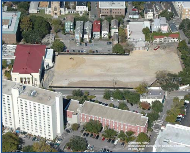
November 2011 - Aerial Photograph Drain Installations Complete
