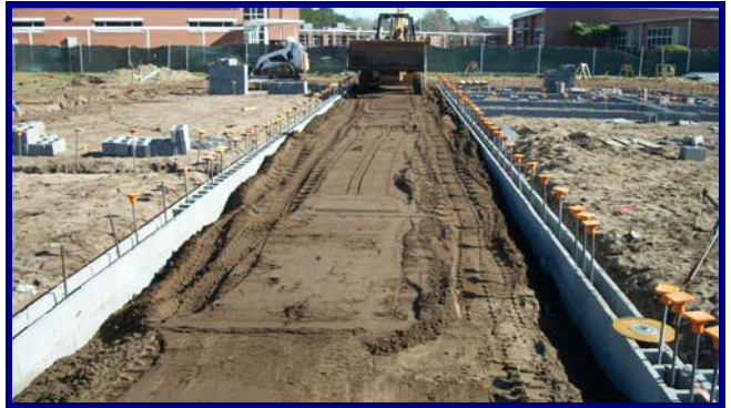
Main Corridor Footings Complete
