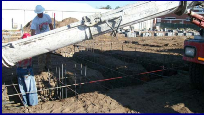
Concrete Placement at Interior Footings
