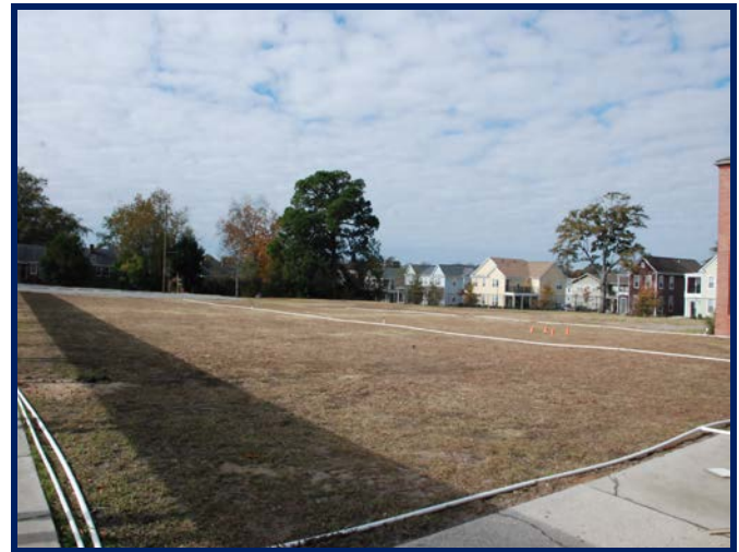
Chicora Move to McNair Campus Grassing and Irrigation at Play Area
