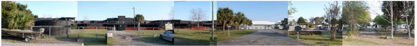
View from Ion Avenue
