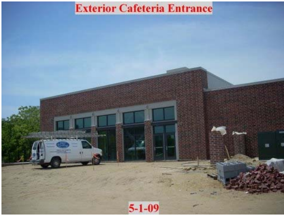
Exterior Cafeteria Entrance
