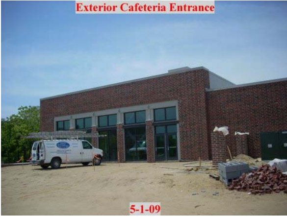
Exterior Cafeteria Entrance
