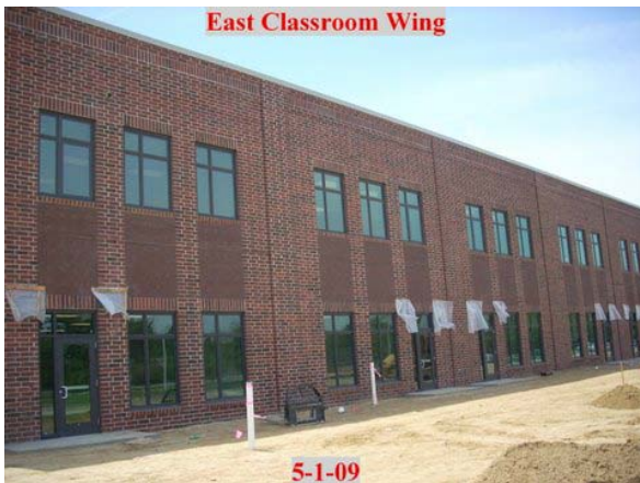
East Classroom Wing
