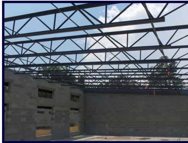
Classroom Roof Joists
