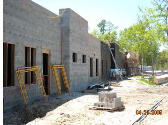
South Wall Wing C
