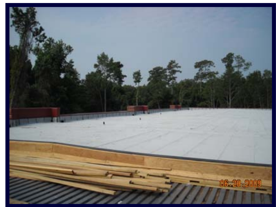
New Roof over Kindergarten
