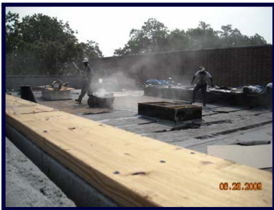
Roofing over Art Room Area
