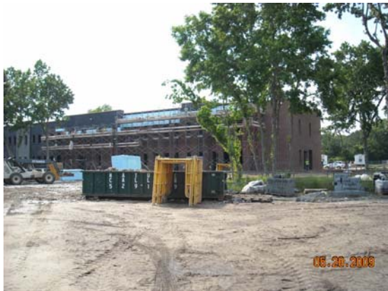
South wall of Area B
