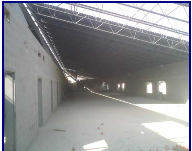
Roof Decking Installations
