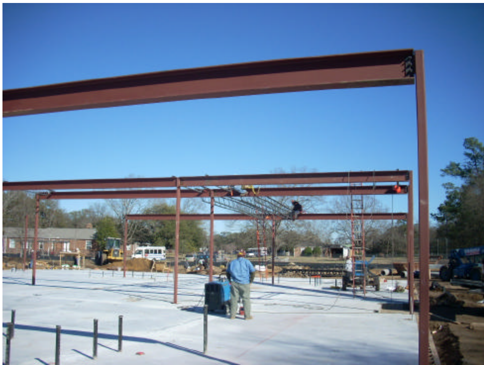
Building Section 1 – Steel Erection
